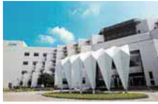
Tainan Plant (Diamond-rated Green Building)
